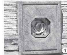
4 Complete placement of manufactured stone veneer or other exterior material around electrical box stone.
